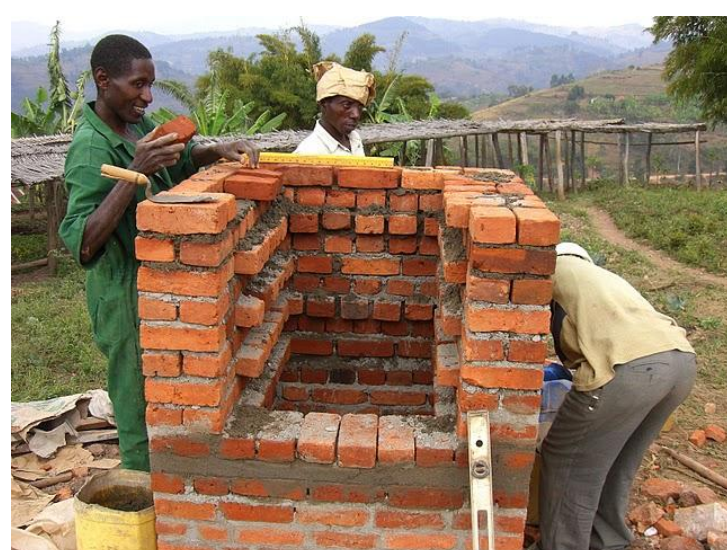
Local workers laying brick for the prototype fruit dryer in Rwanda
